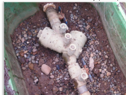
Double Check Valve Assembly (DCVA)
